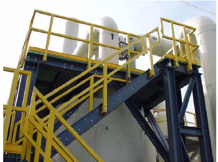
EPP industrial fibreglass handrails are commercial railing systems for stair rails, platform/walkway handrails and guardrails. The EPP systems are fabricated from pultruded fiberglass components and moulded thermoplastic connectors. The railing systems are particularly well-suited to corrosive environments like those found in industrial, chemical and wastewater treatment plants as well as commercial structures with urban and salt air corrosion.
